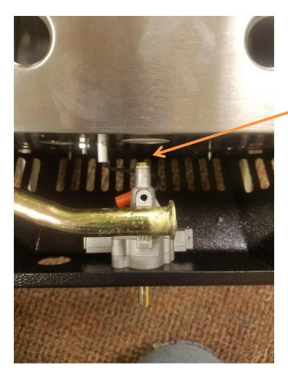
When you install the new burner, make sure the end of the valve is inserted into the burner tube so that the gas goes up into the burner. Then go ahead and screw the burner into place.
